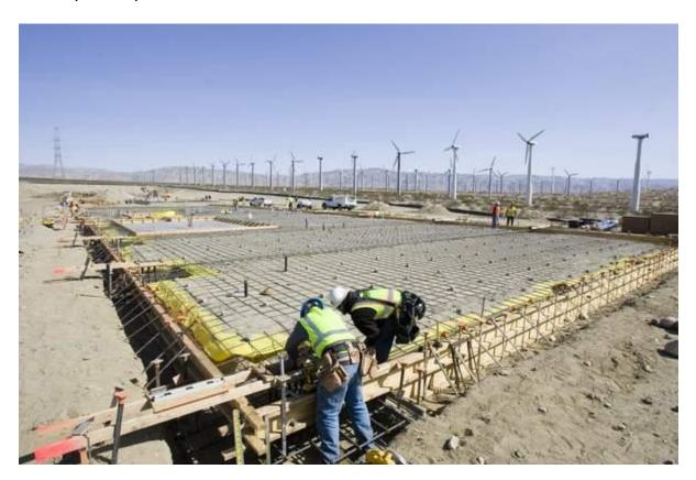
Workers build a foundation at the CPV Sentinel peaker power plant. The plant, which would be able to run up to 116 days a year, will have eight General Electric LMS-100 turbines that each will be able to produce 100 megawatts. / Omar Ornelas, The Desert Sun
